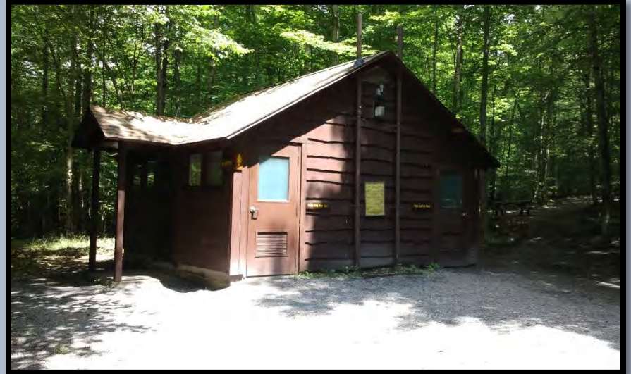
Loop V Comfort Station
