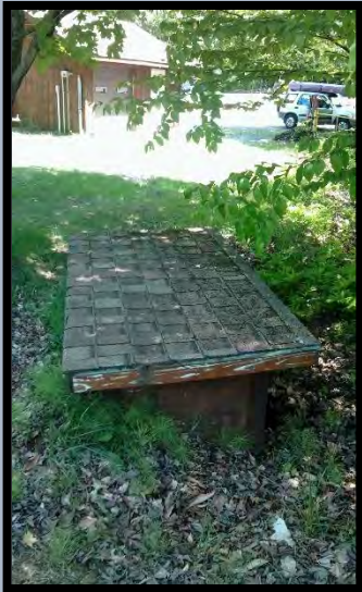
Shower Building Pump
