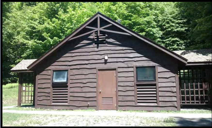
Comfort Station Near Site # 21
