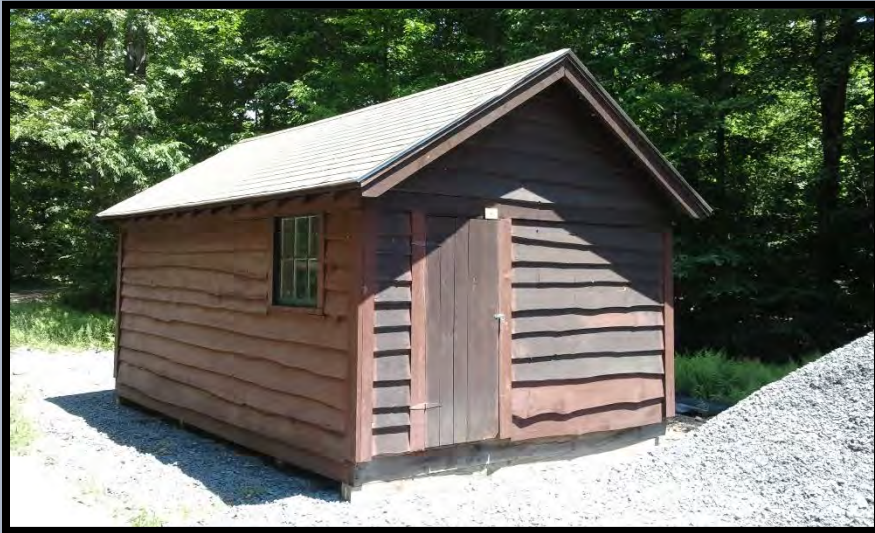
Reservoir Road Storage Building
