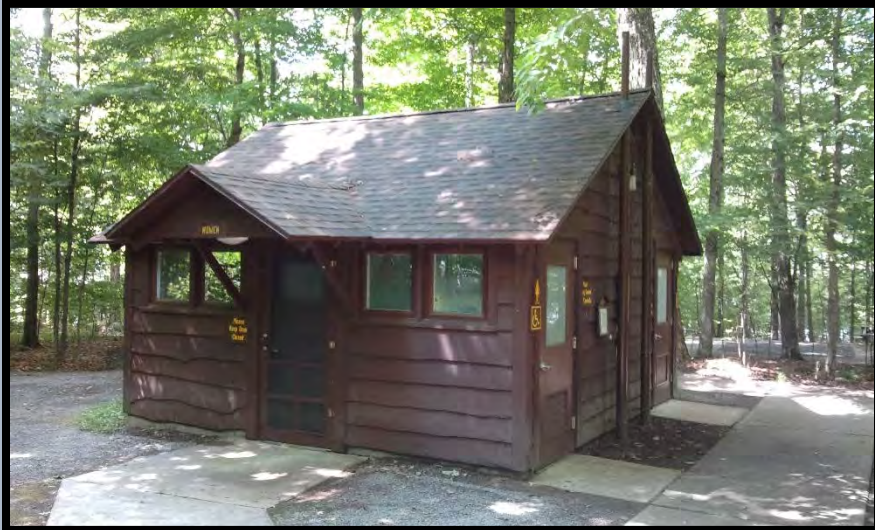
Loop III Comfort Station
