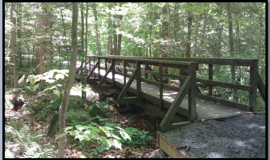
Peninsula Loop Comfort Station Bridge
