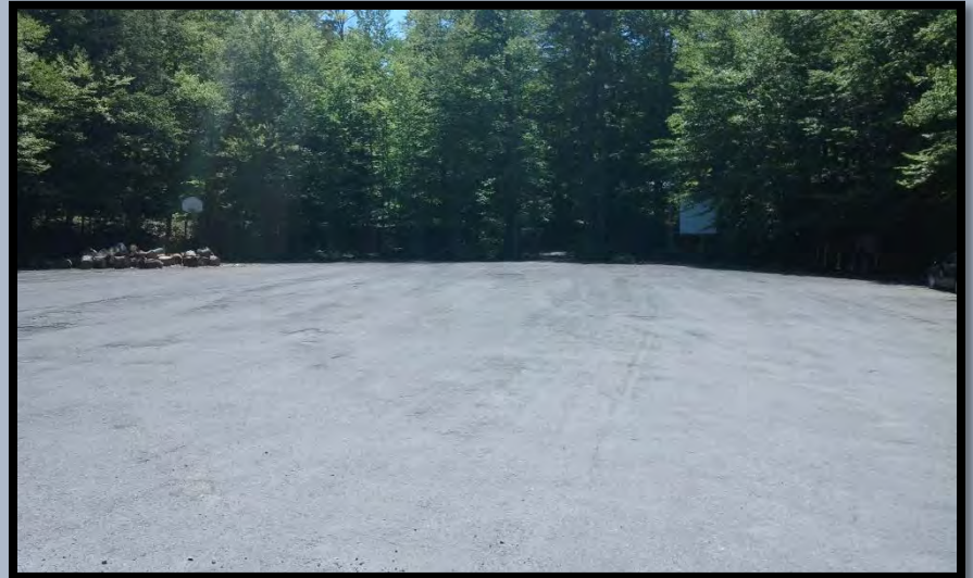
Shower Building/Recycle Center Parking Lot
