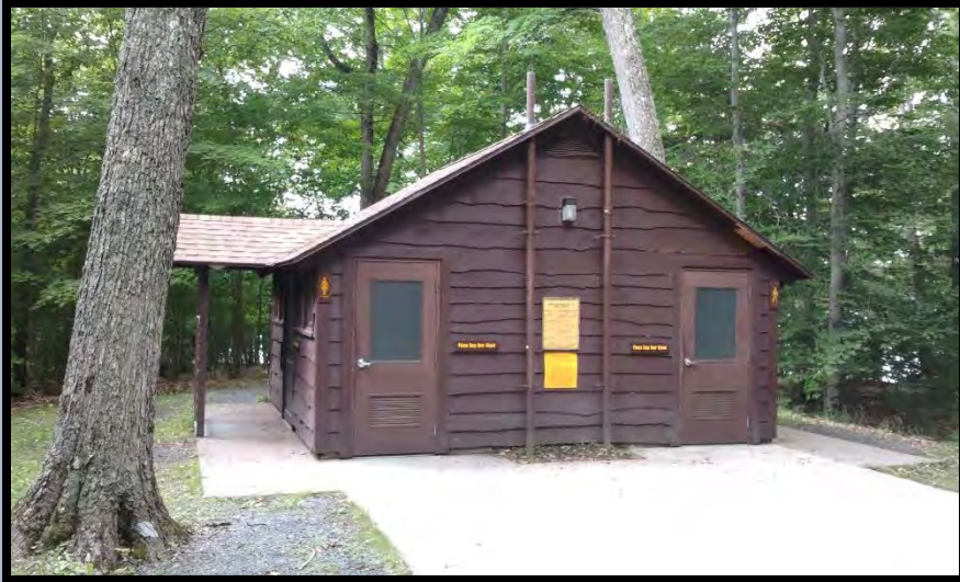
Loop II Comfort Station
