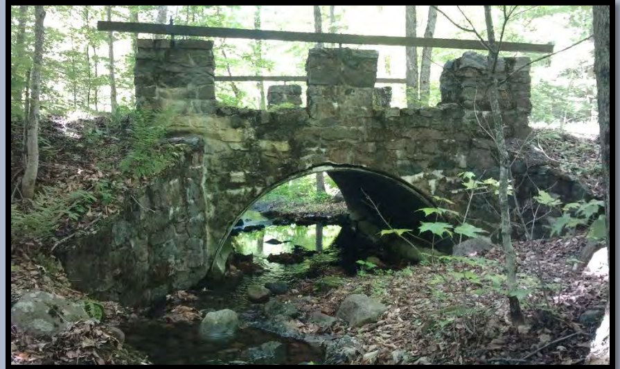
Bridge Near Site #27
