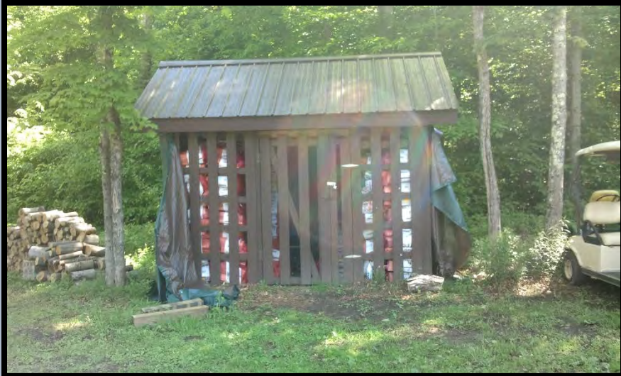
Wood Storage Shed
