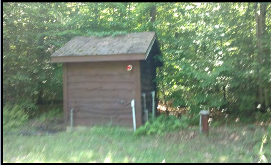
Reservoir Rd. Pump house and Well
